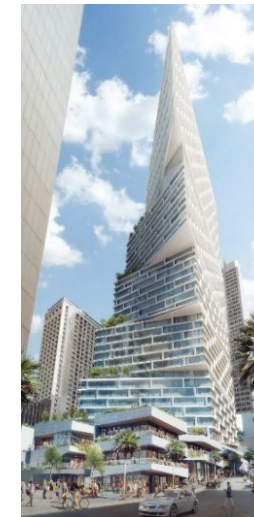
Quay Quarter Tower
